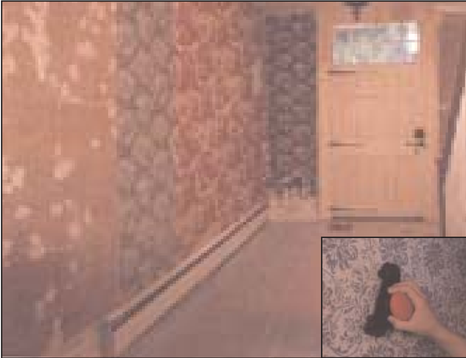
Multiple layers of wallpaper, shown during removal in the entrance hall, were first scored with the Triple-headed PaperTiger Tool (inset) and then sprayed with DIF Wallpaper Stripper as shown in photo of worker in another room, as restoration of the 1805 home proceeded.
