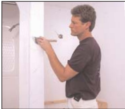
Perma-White, being applied here, is used exclusively in bathrooms by a motel renovator.
