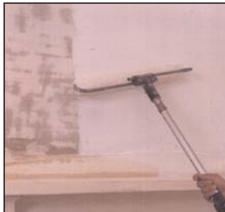
After residual paste was removed with DIF, the walls were primed with Bulls Eye 1-2-3. Ceilings on the second floor were primed with B-I-N, a vapor barrier as well as stain-blocking primer, to keep moisture from damaging attic insulation.
