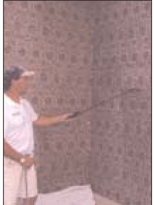
Multiple layers of wallpaper, shown during removal in the entrance hall, were first scored with the Triple-headed PaperTiger Tool (inset) and then sprayed with DIF Wallpaper Stripper as shown in photo of worker in another room, as restoration of the 1805 home proceeded.
