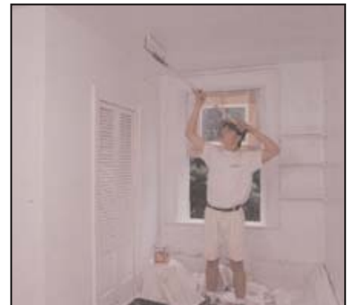
After residual paste was removed with DIF, the walls were primed with Bulls Eye 1-2-3. Ceilings on the second floor were primed with B-I-N, a vapor barrier as well as stain-blocking primer, to keep moisture from damaging attic insulation.
