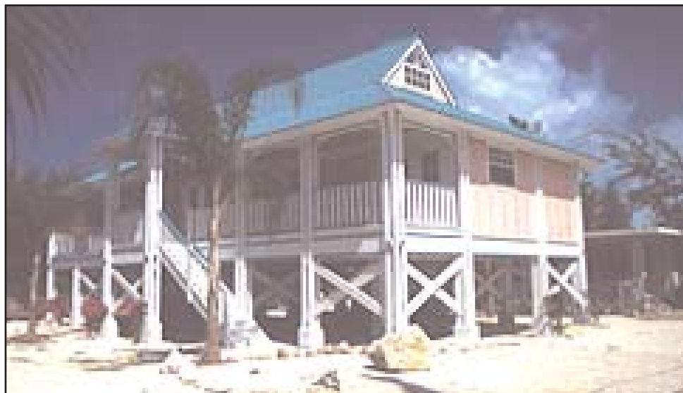
Exterior columns, posts and beams, ornamental trim and handrails of this "Island Style" home were factory-primed with H 2 Oil-Base during manufacture and topcoated on-site when the building was assembled.
